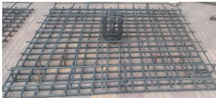
Figure 1 Typical arrangement of slab reinforcement.
